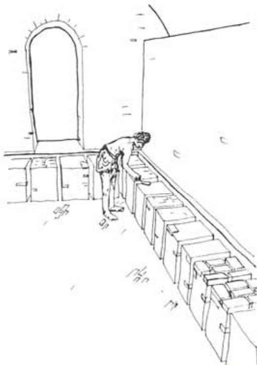
Figure 14: Putting the chequer floor support pillars in the floor of the kiln.
